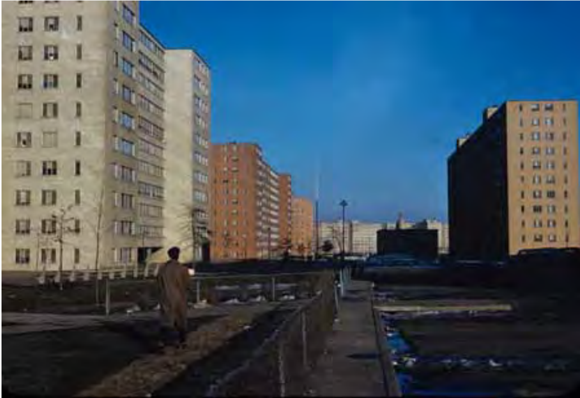
Figure 8 — Identical towers replaced low-rise housing in the final version of Pruitt-Igoe; chain-link fences and thin sidewalks took the place of landscaping and wide pathways. Credit: University of Missouri-St. Louis, Western Historical Manuscript Collection.
