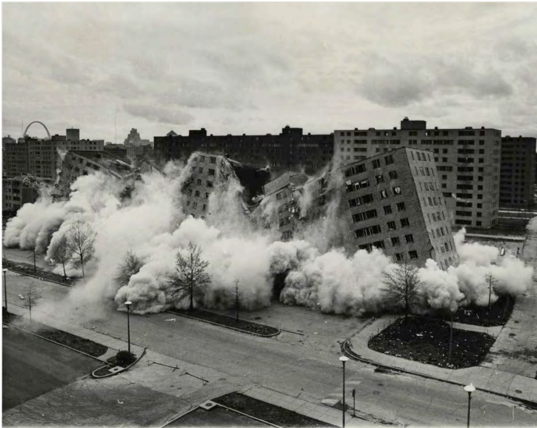
Figure 1 — Signs of decay surrounding the collapsing building are present everywhere: the pavement is buckled and cracked, the grass is littered with debris and garbage, and other buildings are in various stages of demolition in this infamous photograph. Credit: State Historical Society of Missouri, http://www.flickr.com/photos/pruitt-igoe/5472095321/
